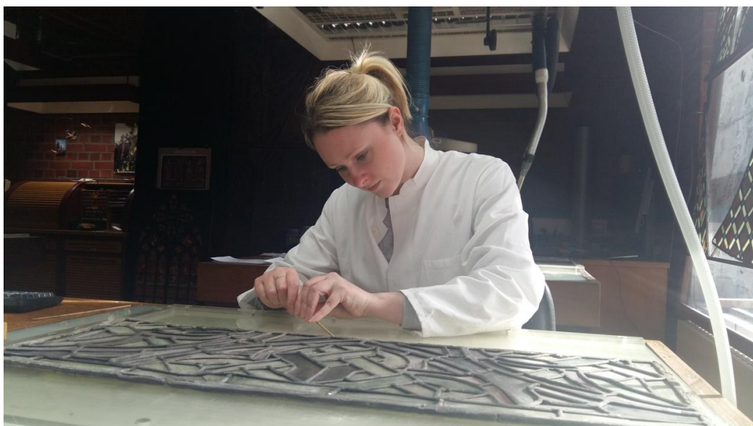
Cleaning the lead matrix of a medieval stained glass panel. June 2016.
